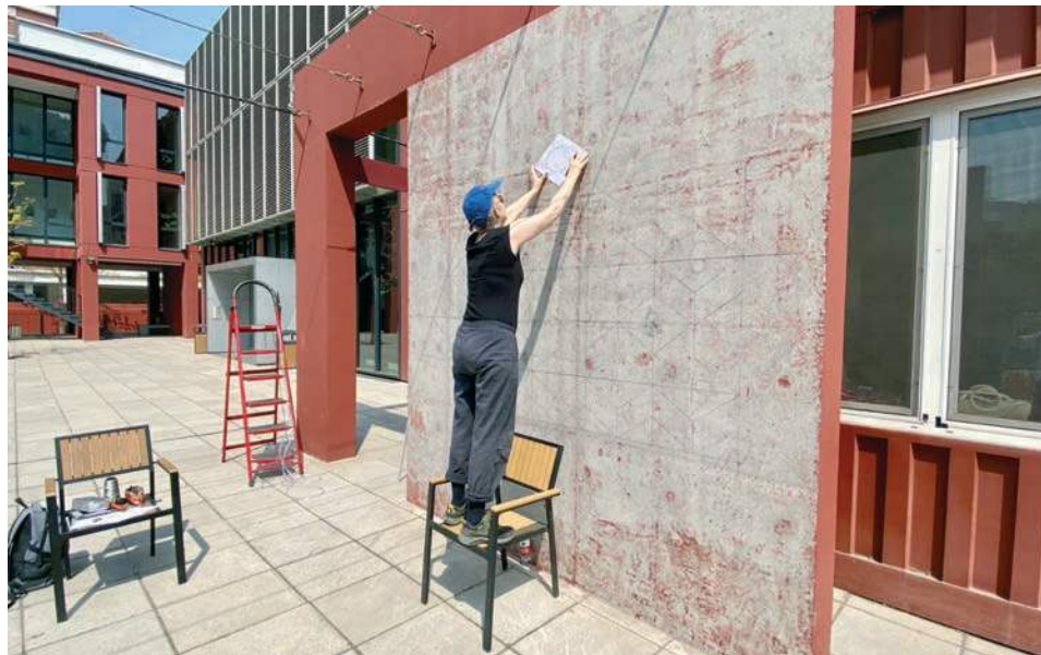
School helpers sand down the wall.
